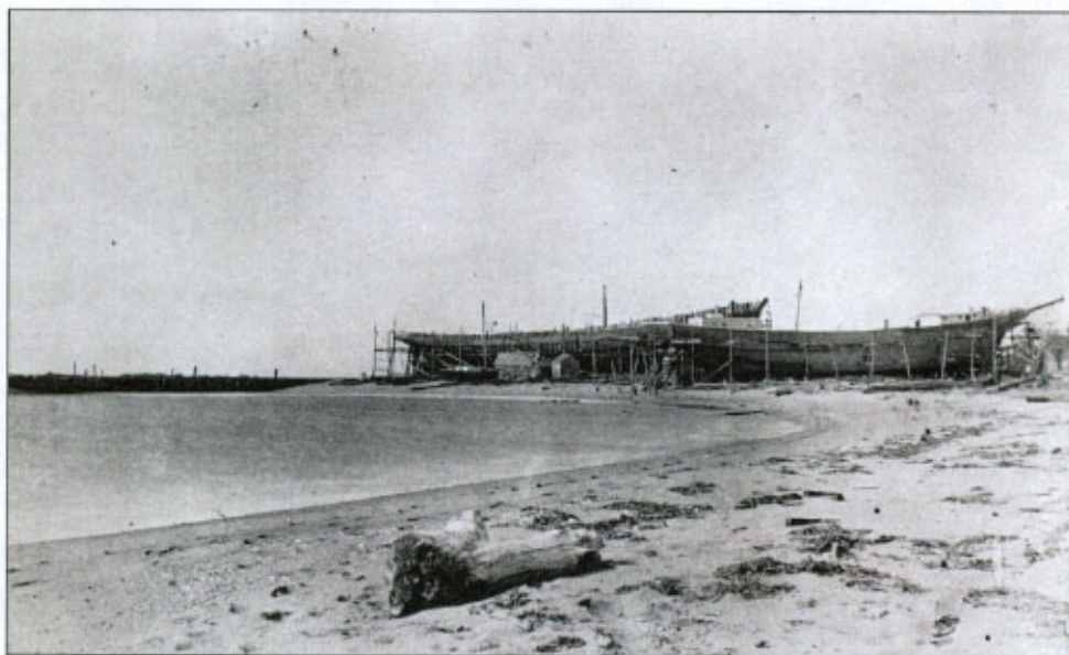
Ships under construction at West Wharf
